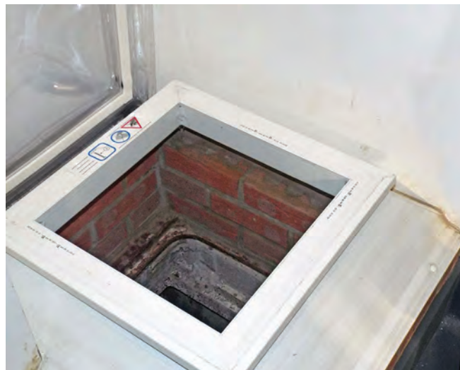
Australia House well access with cover removed. Photo John Lill
